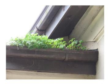
Painted cast-iron and plastic gutters and downpipes - notable amounts of vegetation in gutters.
