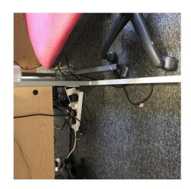
Room F2 - Extension leads used under desks for IT equipement Install additional sockets
