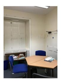
Combination of painted plastered random masonry and lathe and plaster partitions. Generally good to satisfactory with localised areas of plaster defects, presumably linked to historic incidents of water ingress.
