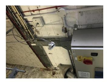
RJ45 outlet hanging loose with bare connections Install surface singlre box and RJ45 mounting plate
