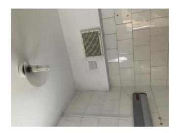
Ground & 1st floor - WC Light broken, Bathroom light not HO batten holder
